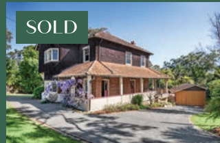
28-32 Beaconsfield Rd, Chatswood
